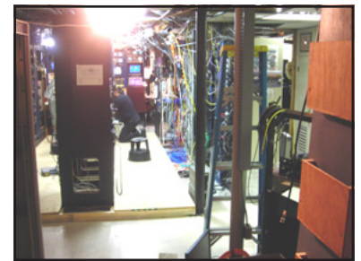
The new master control was built in the middle of the old one as the old one was being dismantled.
